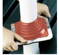
SLIDE... Slide Master Flash down over pipe. (A non-petroleum base lubricant will ease installation.)
